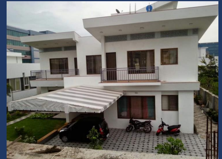
Construction of Bungalow
