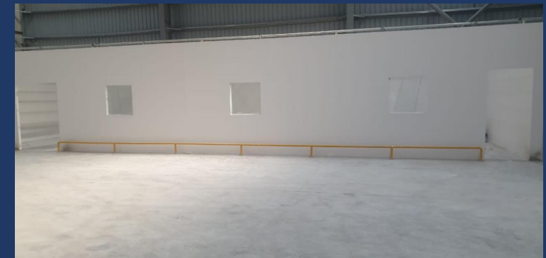
Creation of office space with dry wall partitions for LG Electronics warehouse
