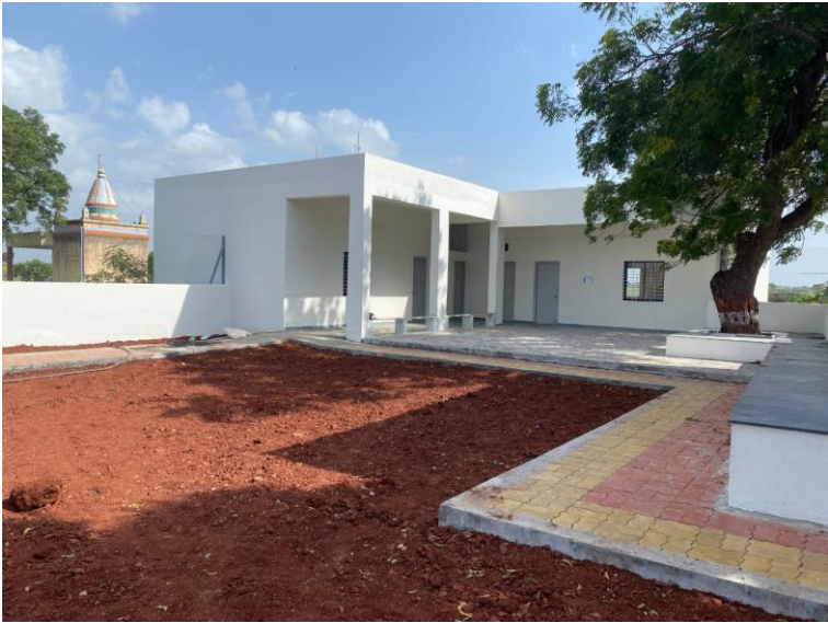
Construction of school building
