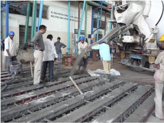
Machine foundation constructed for Kirloskar Pneumatics Ltd, Saswad.
