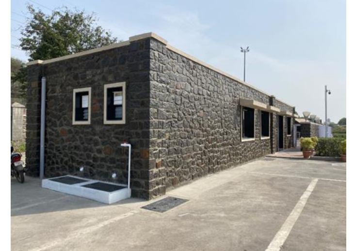
Construction of office building
