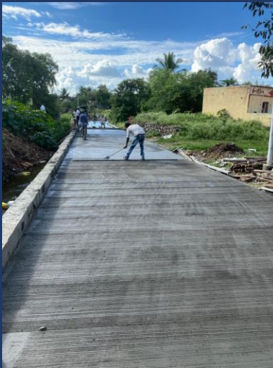
Construction of concrete roads
