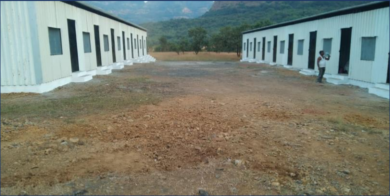
Temporary hutments at Gutke, Tal-Mulshi under CSR activity of Fiat India Automobiles Pvt Ltd
