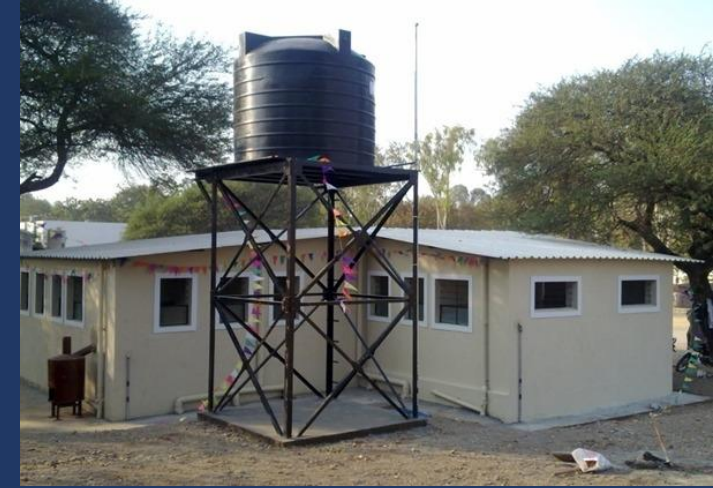
Construction of Toilet blocks under CSR activity for Kirloskar Foundation
