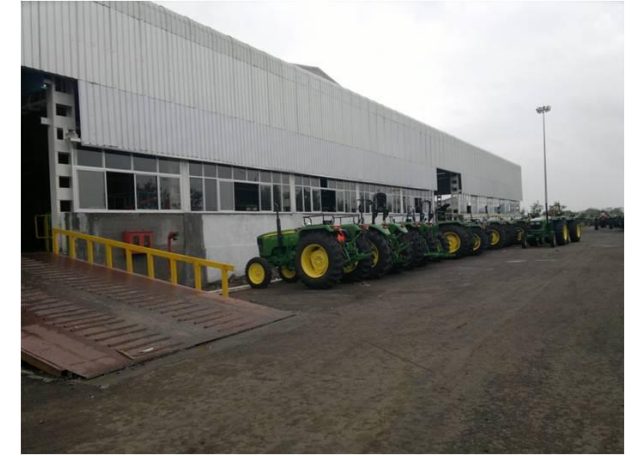
Extension of PDI shed for M/S Johndeer Equipments India Pvt. Ltd. @ Sanaswadi. Area- 1500 Sq.mtr. built in year 2012
