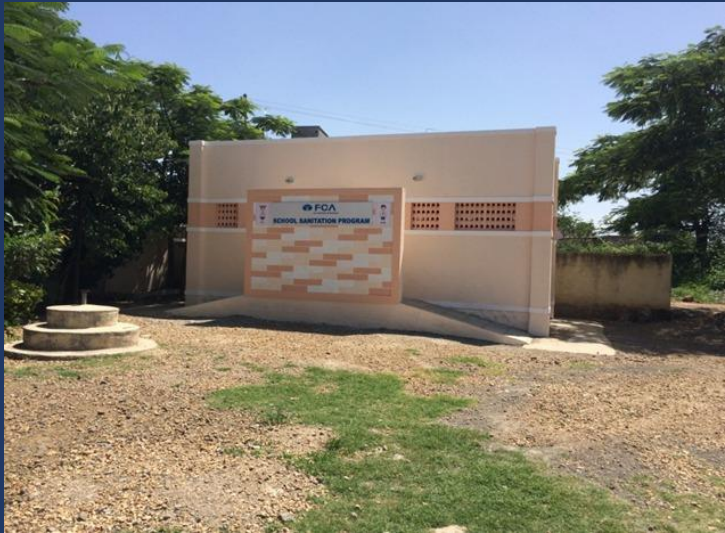
Construction of Toilet blocks under CSR activity for Fiat India Automobiles Pvt Ltd
