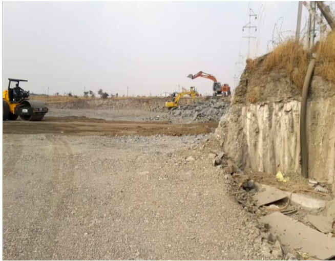
Land Development work of IAC, Chakan
