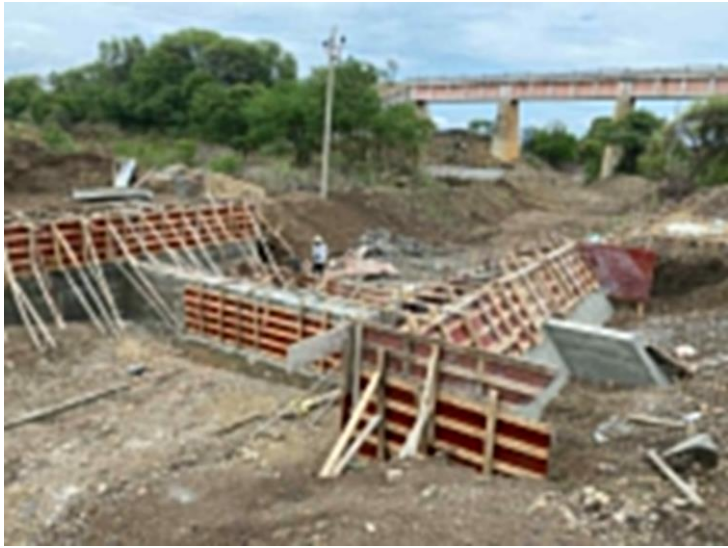
Construction of CNB under CSR activity of Fiat India Automobiles Pvt Ltd, Ranjangaon in Tal-Shirur
