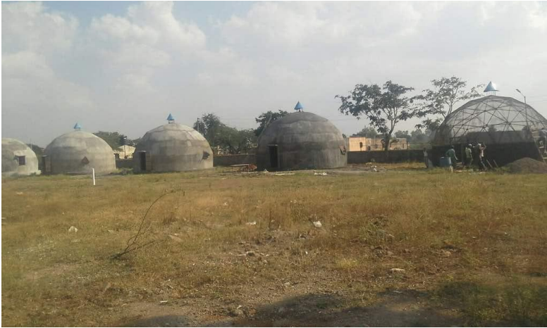
Ferrocrete dome classrooms at Chaufula, Tal-Daund under CSR activity of Cummins Diesel India foundation
